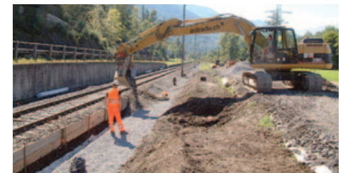
Standard-compliant pipelaying in the drain trench
