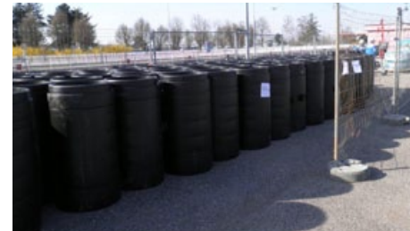
Short-pipe modules, OD = 630 mm x 37.4 mm, at the construction site prior to laying
