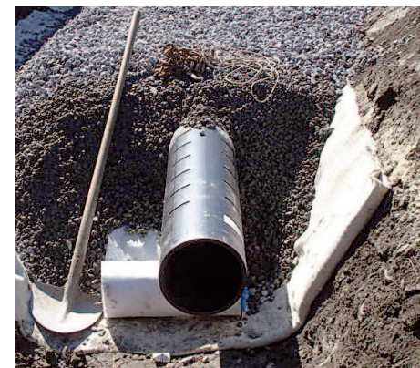
Geotextile jacket round the filter gravel bed
