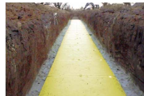
Figure 4: Protective sheets laid over a gas pipeline
