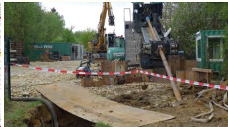
Top: destination pit with jetting tool – product pipe emerging in the destination pit with an attached hole opener; bottom left: the squares mark the locations of wash-boring operations; bottom right: the HDD method is performed by Max Wild, Berkheim, using a silenced 250 t wash-boring rig
