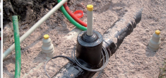
From left to right: Intensive preliminary training ensures a high fabrication quality on the construction site. Connections of hot and cold water pipes. Integrated monitoring systems provide warnings of dangerous leaks.
