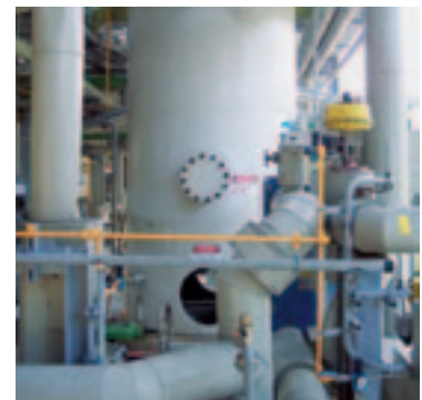
Cylindrical tank made of SIMONA® PVC-C CORZAN Industrial Grade
