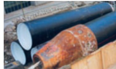
PE 80 coextruded short-pipe modules for insertion using relining method
