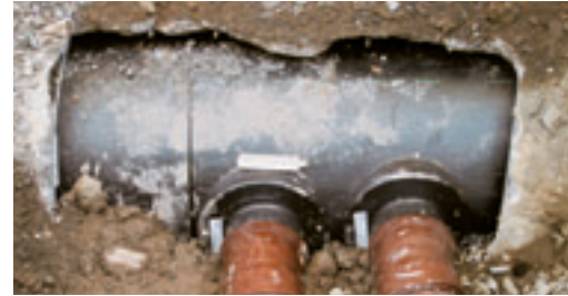
On-site photo: External saddle for service pipe connection
