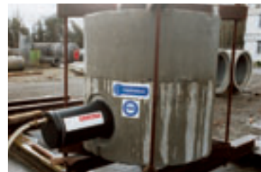
Shaft connection test
