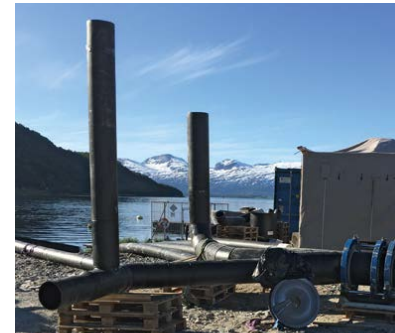
Norway: 12 km of PE 100 pipes and fittings for land-based aquaculture facility
