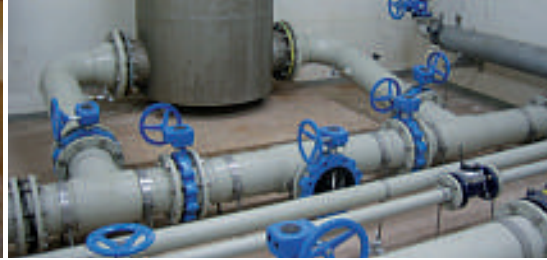
Illustrations from left to right: Corroded joints of the tiled tank; PP-H 100 AlphaPlus piping system in the pre-chamber; pump sump with discharge strainer
