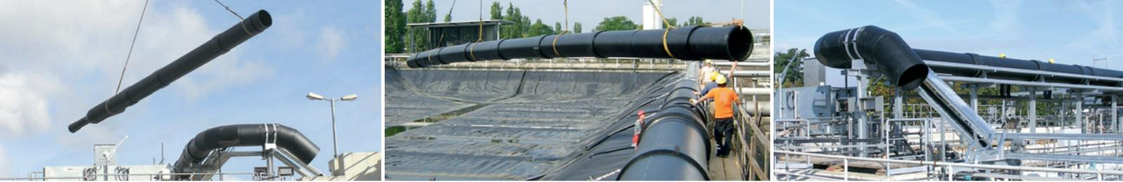
Fig. from left to right: A250-ton mobile crane with a maximum radius of 70 metres effortlessly lifts the individual elements. Pre-welded pipe elements help to reduce the overall assembly time.
