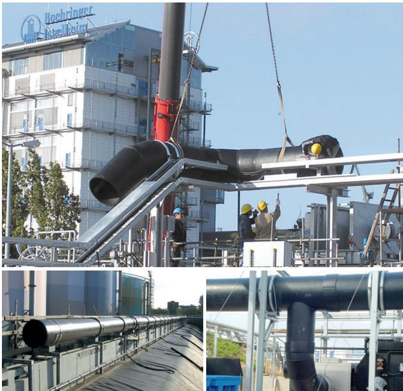
*The pipes are securely supported on a network of pipe bridges. Numerous special components enable individual adaptation to the local conditions.*
