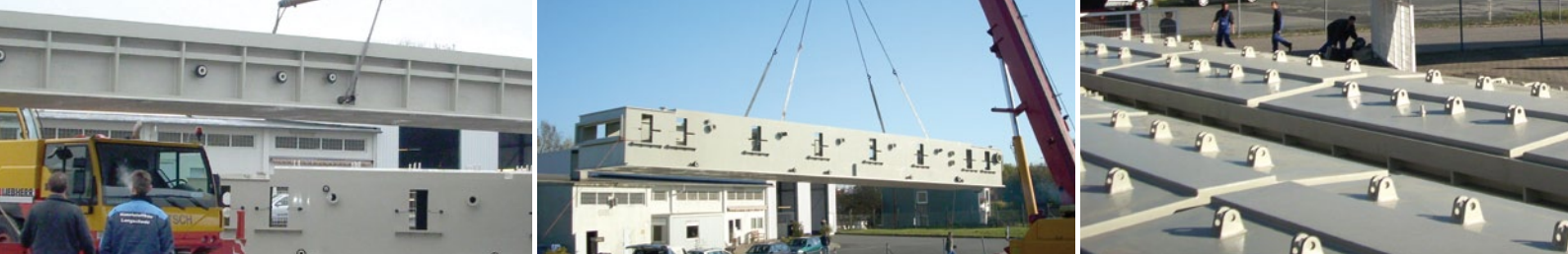
Delivery of the pickling tanks to the Rasselstein steel plant
