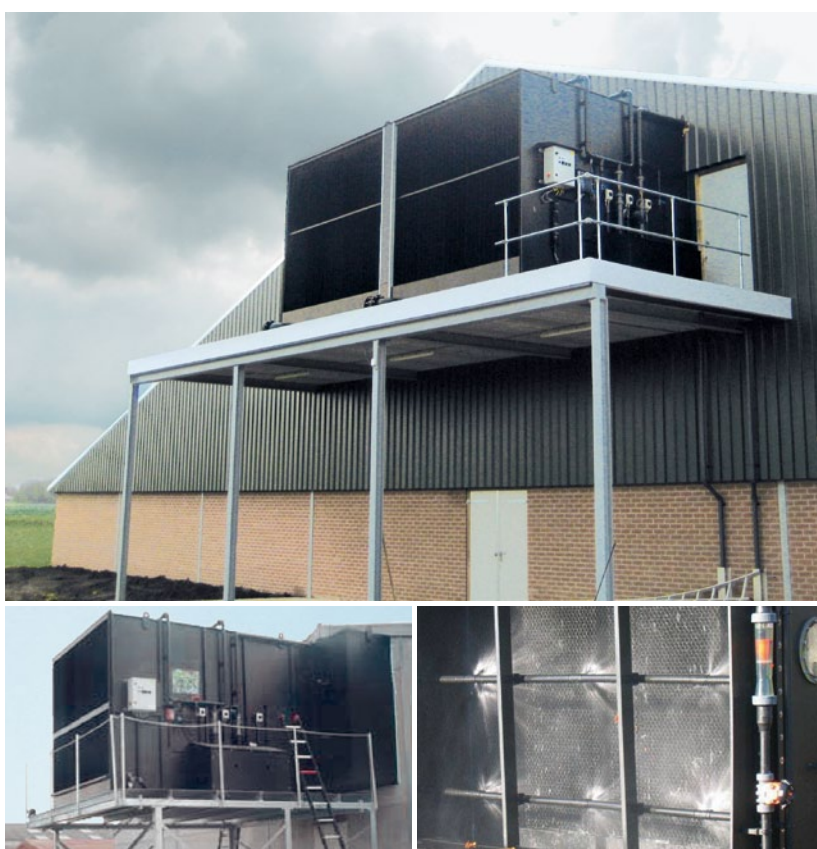
Top/bottom left: outdoor Nitro Air scrubber developed by KWB, Netherlands; Bottom right: Nitro Air scrubber in use
