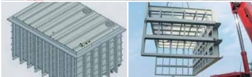
Top: completion of the tank; bottom left: design drawing with steel basket; bottom right: loading part of the steel reinforcement
