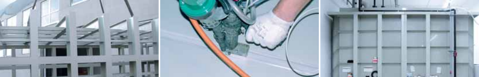
From left to right: part of the steel reinforcement; welding the tank on site; tank in the installation
