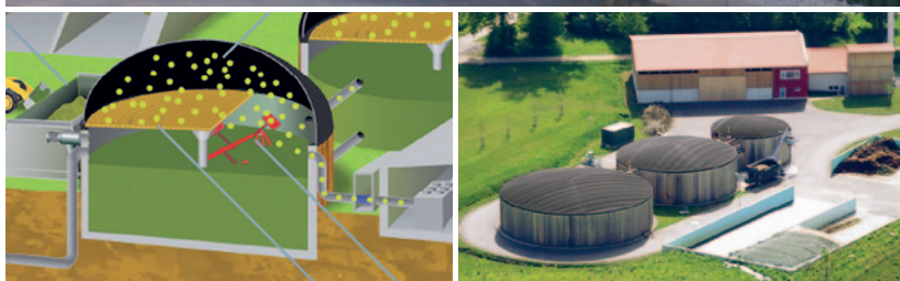
Top: view of the fermenter and secondary fermenter; bottom left: diagram of how the biogas plant works; bottom right: biogas plant completed
