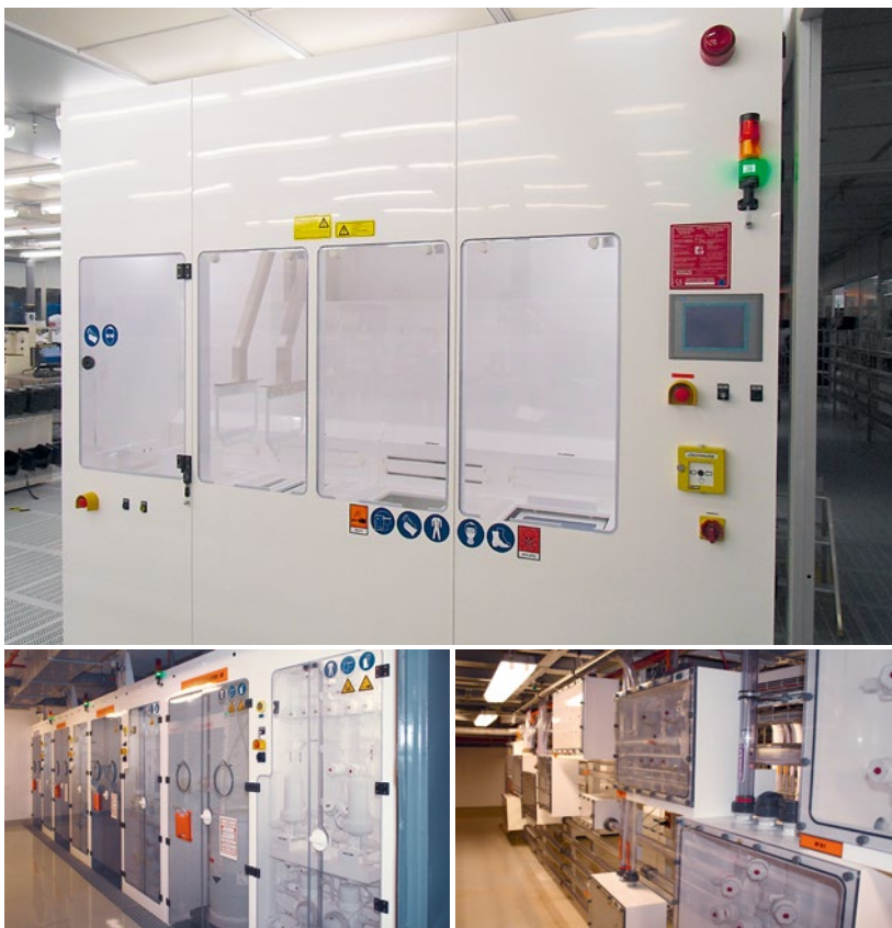
Top: automated wet-processing unit for the machining of silicon wafers; bottom left: fully automated supply systems for high-purity chemicals; bottom right: distribution systems for equipment ports
