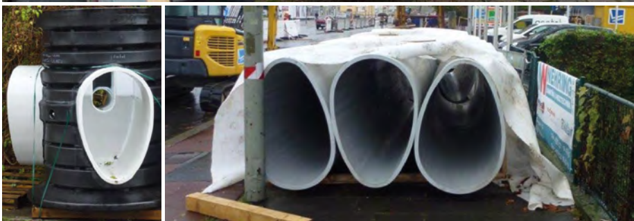
Top: two welded ovoid pipe modules with socket band fitted; bottom left: CoEx shaft with light-coloured inner layer and ovoid pipe connection; bottom right: storage of the ovoid pipes without a base on the construction site
