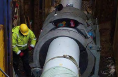
From left to right: factory pre-welded ovoid pipe trains undergoing the client's welding and cooling process in a welding machine; ovoid pipe without base in the open trench; special aspect of geometry leads to excellent discharge characteristics depending on the level of sewage in the pipe
