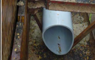
From left to right: factory pre-welded ovoid pipe trains undergoing the client's welding and cooling process in a welding machine; ovoid pipe without base in the open trench; special aspect of geometry leads to excellent discharge characteristics depending on the level of sewage in the pipe
