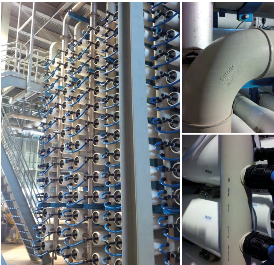
Left: view of distribution system – customised design consisting of pipes, fittings and flanges with required pressure ratings; top right: SIMONA® injection-moulded bends possess very good hydraulic properties; bottom right: SIMONA® PP-H AlphaPlus® Pipe with outlet points in requisite pressure ratings
