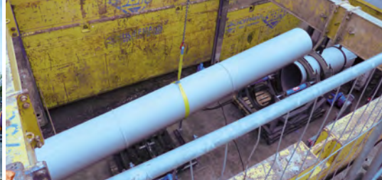
From left to right: introduction of the factory-welded 7.5 m module to the trench and welding it to the pipe train for relining insertion
