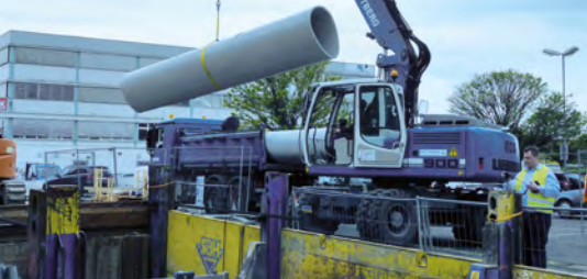
From left to right: introduction of the factory-welded 7.5 m module to the trench and welding it to the pipe train for relining insertion
