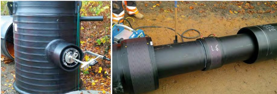
Top: Factory-prefabricated SIMONA® PE 100 Pressure Pipe Shaft with double-containment pipe connections and preparation for accommodation of a leak detection unit; bottom left: Peeler from the SIMONA® tool hire facility; bottom right: Cascade welding of the SIMONA® Double-Containment Pipe d = 355/500 mm
