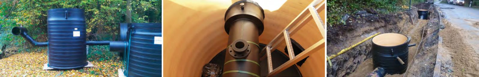
From left to right: Factory-prefabricated SIMONA® PE 100 Pressure Pipe Shafts; view inside the shaft with double-containment pipe to single-pipe adaptor and reduced tee for accommodating the ventilation unit; pressure pipe shafts and double-containment pipe laid in the open trench
