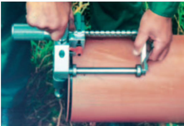
Preparing the pipe ends for heating element butt welding. The protective jacket is only removed from the welding zone.
