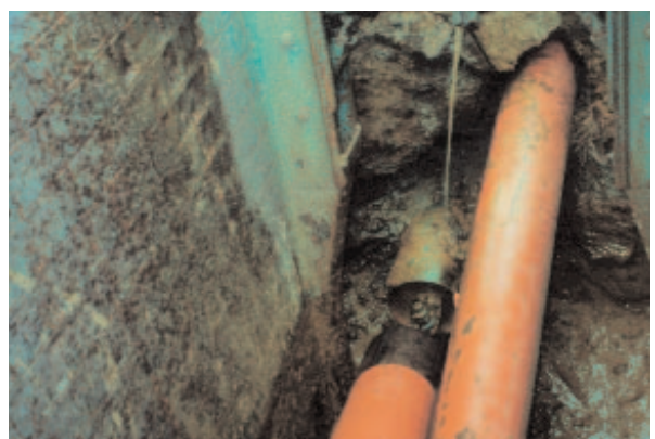
Flush head before pulling into the ground (left: pipe to be installed, right: old pipe)
