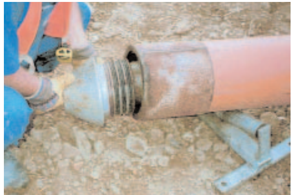
Attaching the pulling head to the SIMONA® SPC protective-jacket pipe
