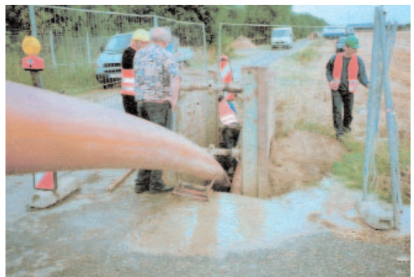
Pulling the pipes for installation via the launch shaft
