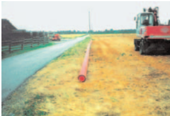
Pre-welded piping prepared for installation
