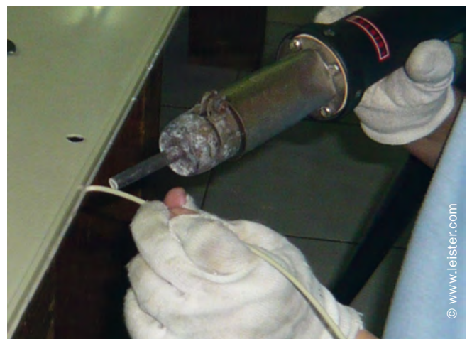
Figure 4: Hot-gas fan welding with circular welding rod
